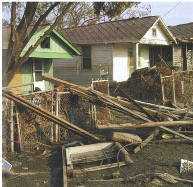
HARD HIT: Hurricane Katrina's devastation shows the need for tougher building standards.
