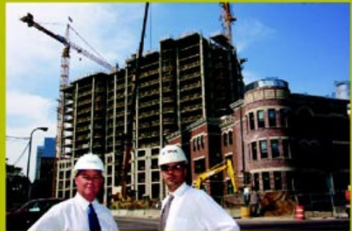
Grant Park- under construction
