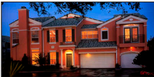
Photo courtesy of Humphreys & Partners Architects
