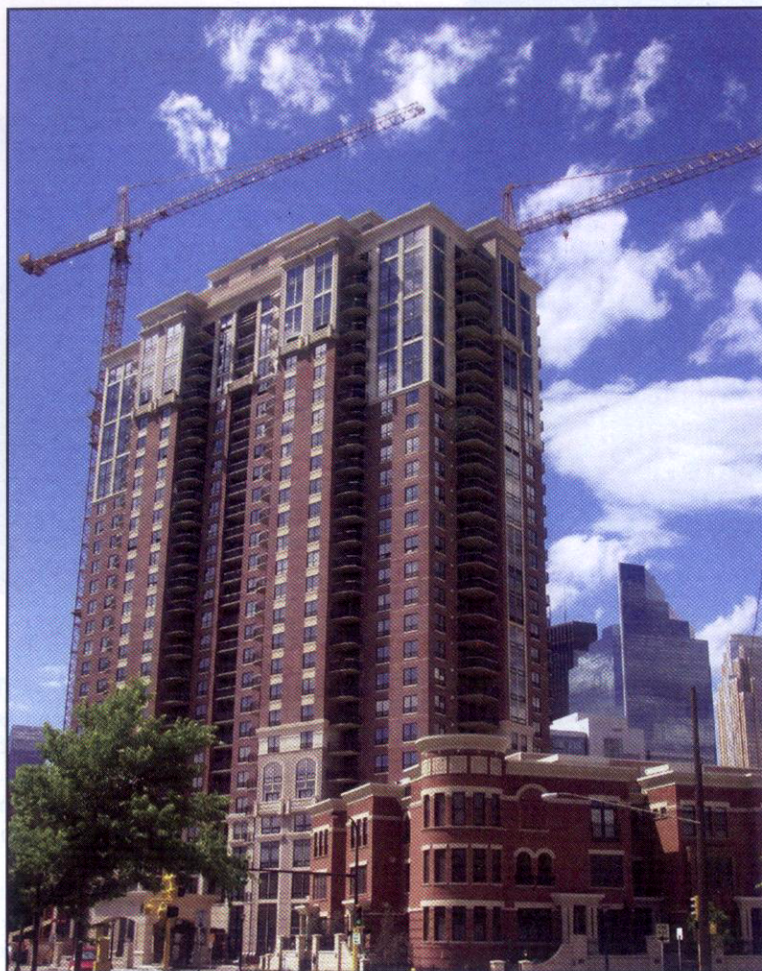
Grant Park in Minneapolis, Minn., is a 27-story, 330-unit development that was staged in four areas: townhomes, tower, garage, and staging/final phase.
