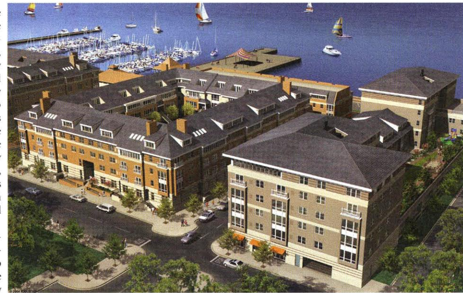
The Landings at HarborSide will add 22 buildings to Perth Amboy, N.J., as well as retail, a waterfront promenade and parks. The design challenge was to create an entire community that holds together aesthetically, isn't repetitious and links the greater community to the city of Perth Amboy.
