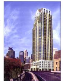
The Carlyle—Minneapolis, MN 39-story Condominium Tower; 280 units Tunnel Form Construction
