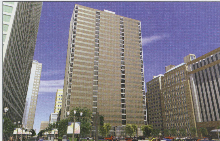
Rockwood Realty Associates is transforming the 1200 Main office skyscraper in downtown Dallas into The Metropolitan, a 283-unit, $50 million condominium project.
