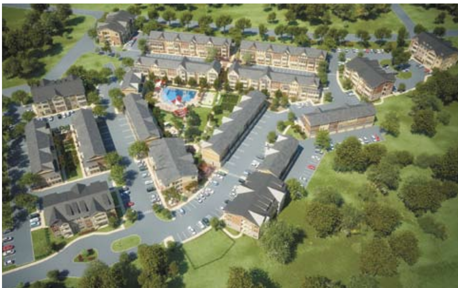
Carter and Associates has broken ground on Tetro Student Village, a 198-unit apartment complex in San Antonio. The property will serve UT San Antonio, which has grown by 68 percent in the last 15 years, according to the school's website.
